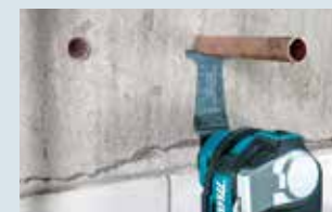
Copper pipe flush cutting
