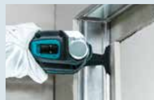
Door opening work
