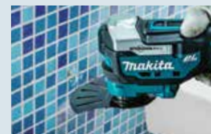
Routing joints on wall tiles
