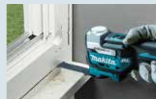
Removal of window frame
